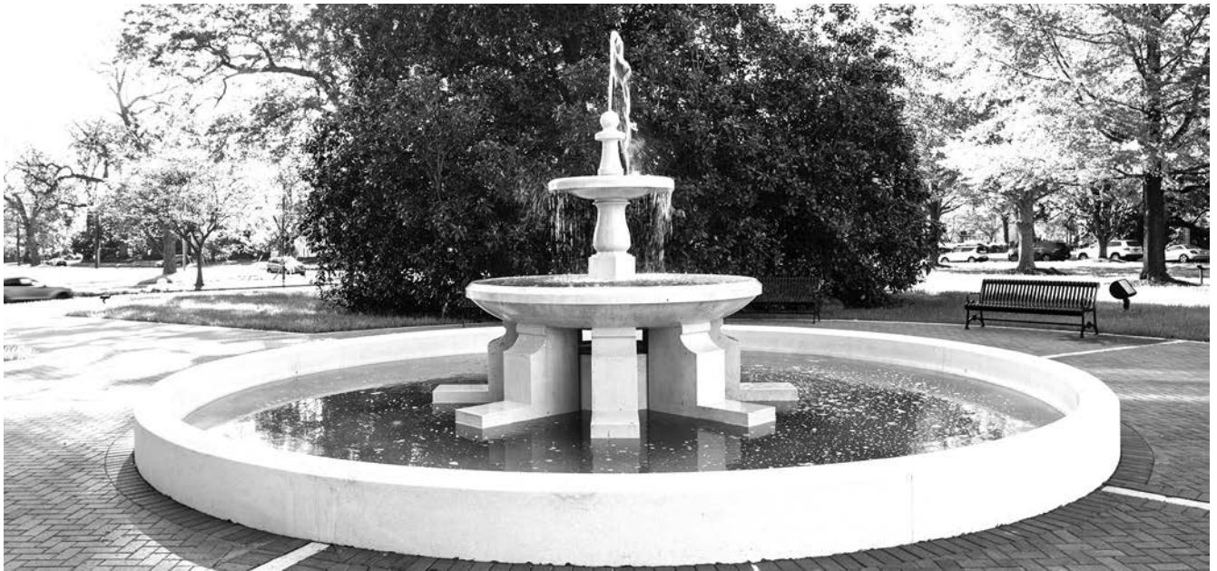
The front campus fountain has served as a popular Winthrop symbol since it was constructed in 1912. It was completely reconstructed in 2023.
