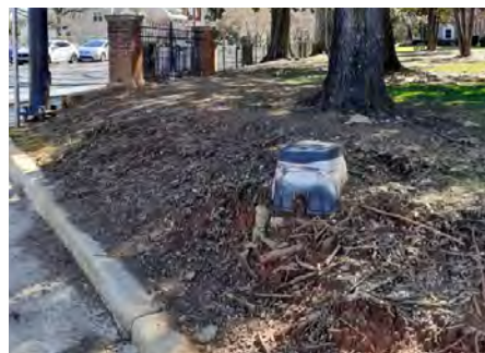
Poor Presentation - Oakland Entrance
