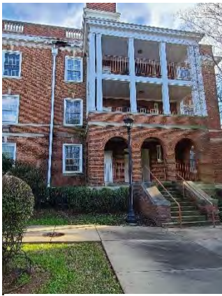
Power wash, Repair - Roddey
