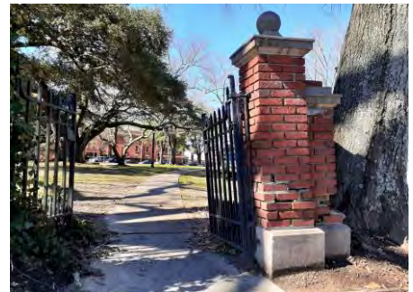
Repair Bricks - Main Administration Building Loop Entrance
