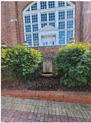
Opportunity - Windows, Walls
