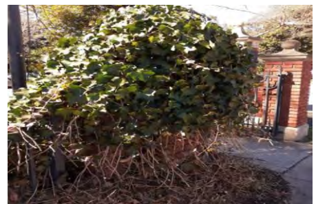
Overgrown Ivy - Main Administration Building Loop Entrance
