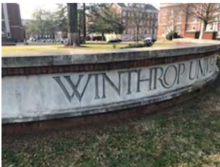
Power wash - Main Entrance Sign
