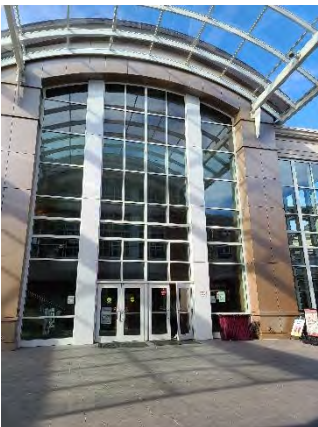
Opportunity - Windows, Walls
