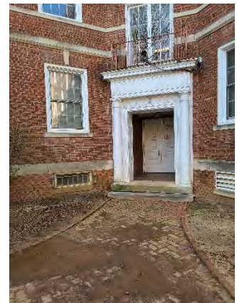
Clean, Light - Roddey Courtyard
