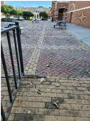
Power wash - West Center
