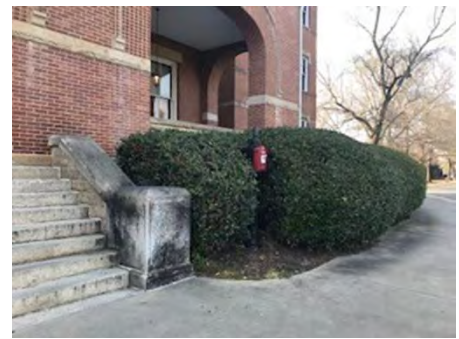
Overgrown Shrubs - Main Administration Building
