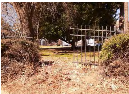
Broken Fence - Johnson Hall Entrance
