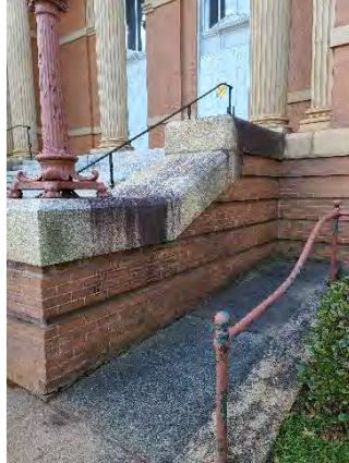
Power wash, Paint - Rutledge
