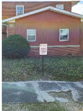
Repair - Sykes House
