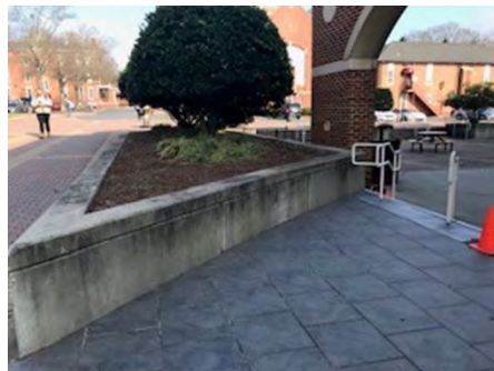
Planting Bed Bare - West Center
