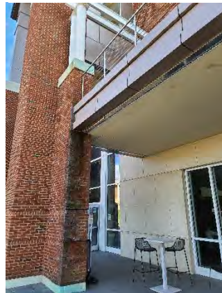
Repair, Paint - DiGs
